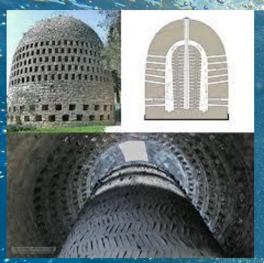
An air well or aerial well is a structure or device that collects water by promoting the condensation of moisture from air. Designs for air wells are many and varied, but the simplest designs are completely passive, require no external energy source and have few, if any, moving parts.
