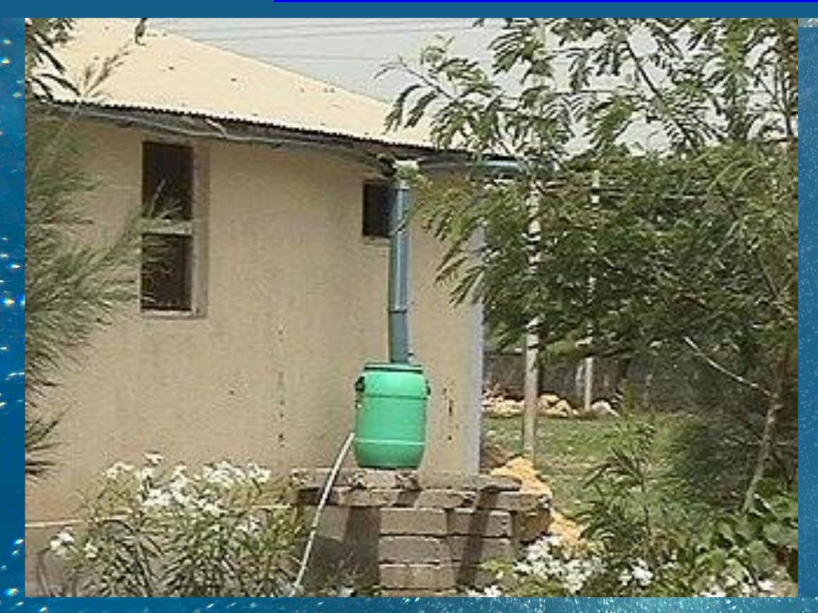
Structures with metal roofing, such as this one, can be used to harvest dew water simply by adding gutters and, for increased output, a layer of insulation underside. without the insulation the output is nearly half of that from plastic condensers.
